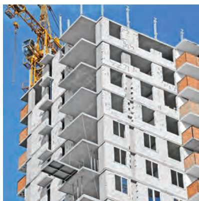
Perimeter walls in carcass building
